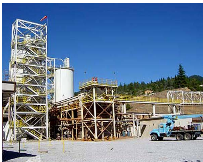
Photo 4: The lime neutralization/high-density sludge acid mine drainage treatment facility at Minnesota Flats.
