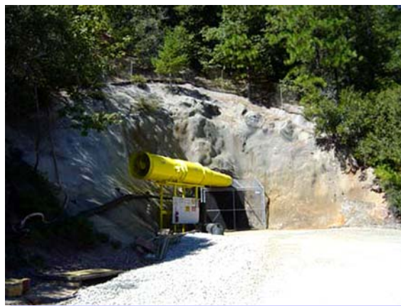
Photo 2: Entrance to the refurbished Richmond adit, showing the ventilation exhaust system.
