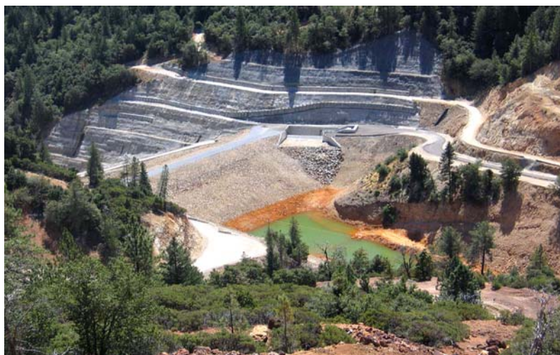
Photo 9: The recently completed Slickrock Creek Dam captures acid mine drainage escaping from fractured bedrock and buried mine portals along the south side of Iron Mountain. The water in the reservoir is transported by pipeline to the treatment plant at Minnesota Flats.
